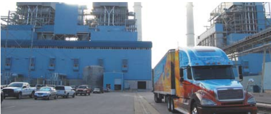
Clyde Bergemann Americas technology trailer at the Fayette power plant
